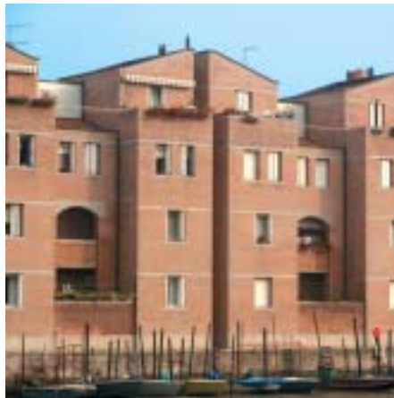
GINO VALLE GIUDECCA - Residential complex IACP (1980-1986), former cement factory
