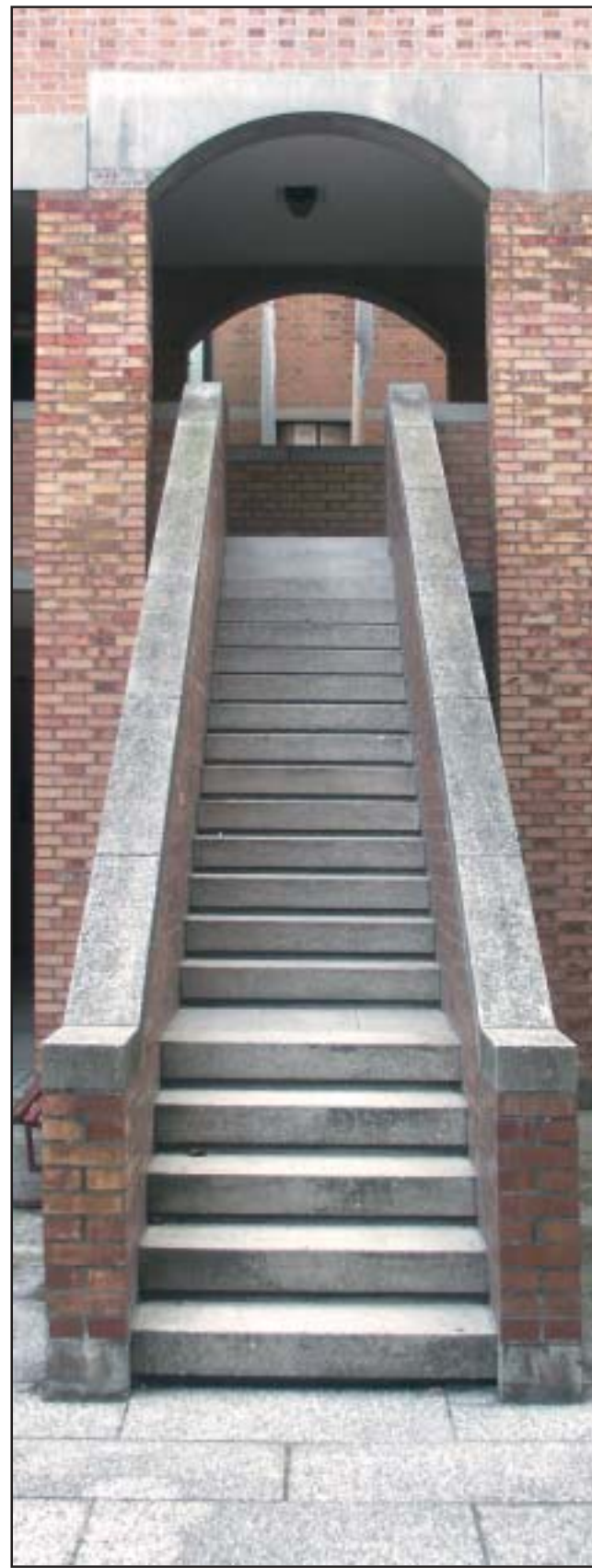
Main stairs of the residential complex Iacp by Gino Valle
